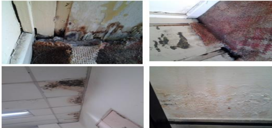
Figure 1. Visible Mould Growth
