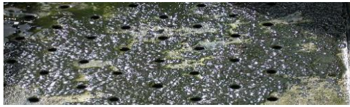
Figure 6a: Algae on Cooling Tower Fins
