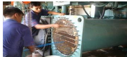
Figure8: Water Being Flush Out During Tubing Cleaning Works
