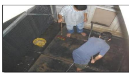
Figure 10: Cleaning Cooling Tower Hot Basin
