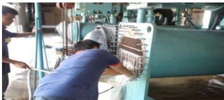
Figure 7: Tubing Cleaning Tubing Cleaning Works
