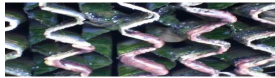
Figure 6b: Algae on Cooling Tower Hot Basin Micro Biological Attack
