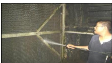
Figure 9: Cleaning Cooling Tower Fins
