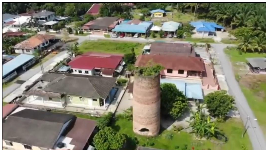
Figure 1: The Japanese Carbide Chimney on the right at Kampung Tanjong Bakong, Malim Nawar, Perak
