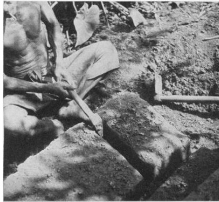
Figure 12: Manually cut laterite using pickaxe in Chanburi, Thailand Source: Pendleton (1940)
