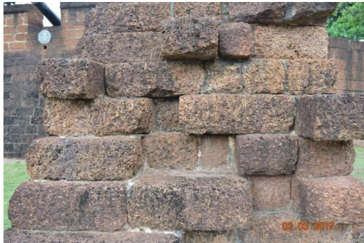
Figure 6: Bastion Middleburg, Melaka-laterite blocks, cemented with concrete and mortars Source: Authors, 2018.
