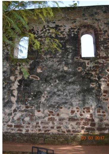
Figure 9: St. Paul's Church, Melaka-seaward wall of laterite stone materials
