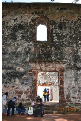
Figure 10: St. Paul's Church, Melaka-detail of side door frame on seaward side wall using laterite stones
